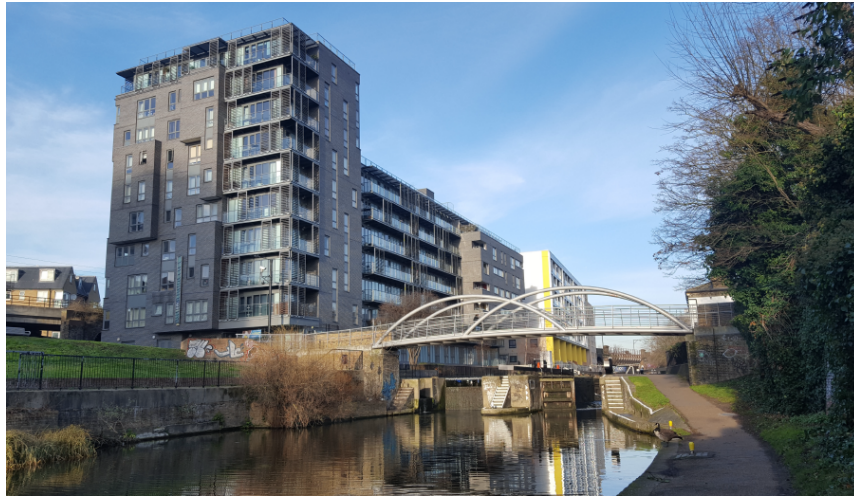
Photograph of the development opposite the site.
